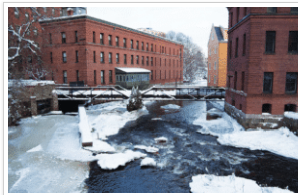
Dorchester Lower Mills, on the Boston-Milton line and next to areas Milton officials rezoned this month to comply with the MBTA Communities law. iStock photo
